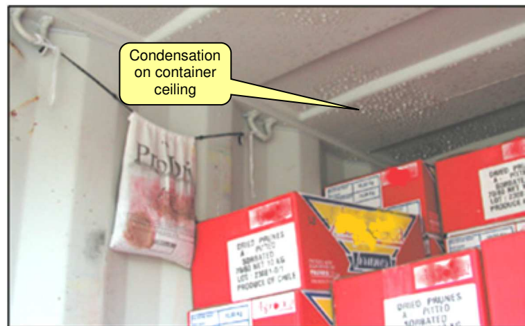
Figure 39-A – Condensed moisture in the container ceiling
